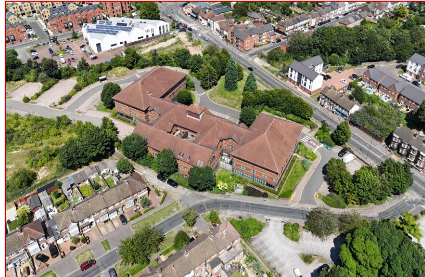
Watling House South Elevation
